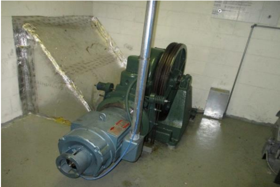
19 Elevator Motor Overview
